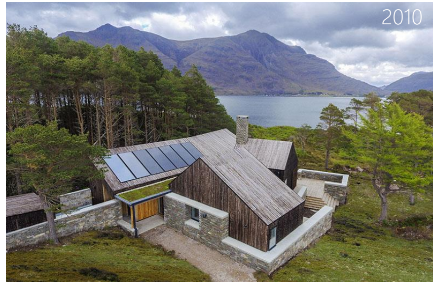
Clearline PV Roof integrated solar photovoltaic panels
