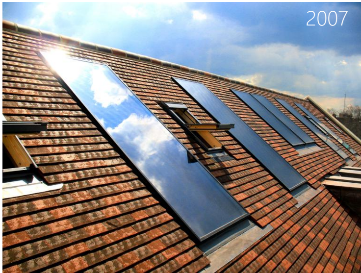
Clearline Roof integrated solar thermal panels
